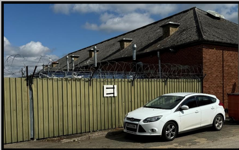
Existing Fence Line
