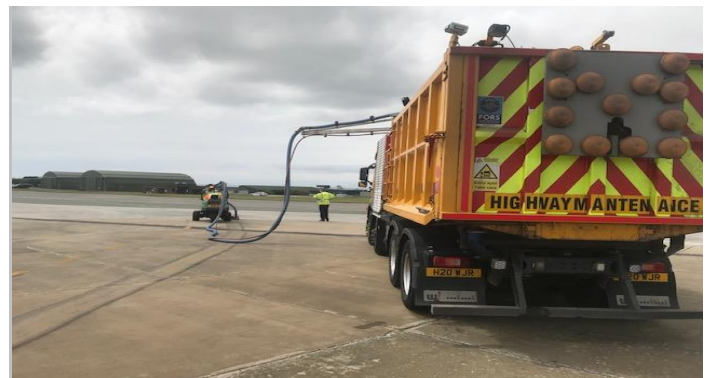
Operating Hydro-blasting Units
