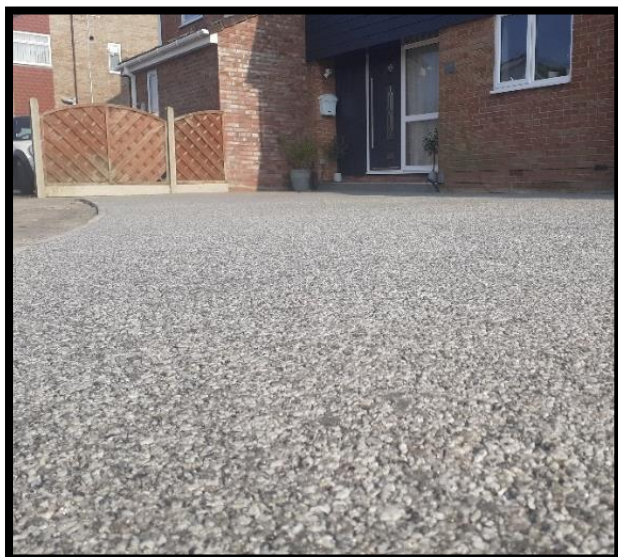
6mm Stirling Silver SureSet being laid over an open graded binder course layer.
